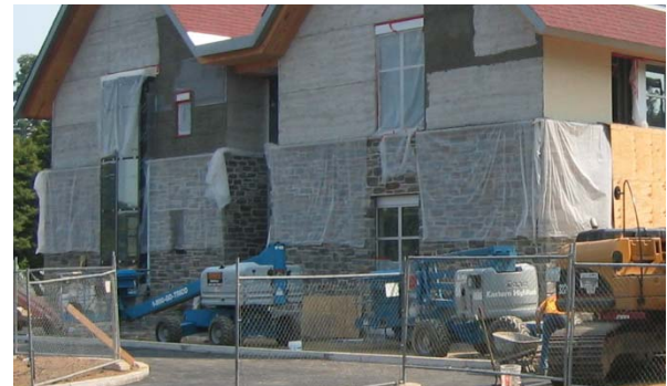
Field Stone Facade & Stucco Construction
