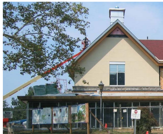
Figure 1 Worker using lift for roof access
